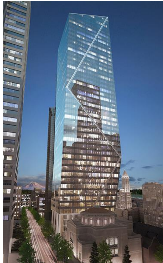
The Mark expands as it rises and cantilevers over the neighboring church, but a trick of the eye in the design will make it sit gracefully on the narrow lot.
