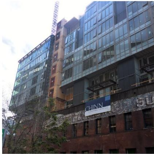
The Gridiron under construction in August 2017. | Sarah Anne Lloyd
