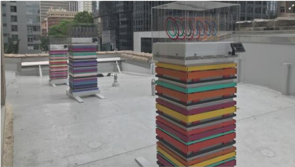
The custom multi-colored hives on the roof of the Sanctuary at the Mark in Seattle are designed by ZGF Architects, the firm that designed the adjoining F5 Tower.
